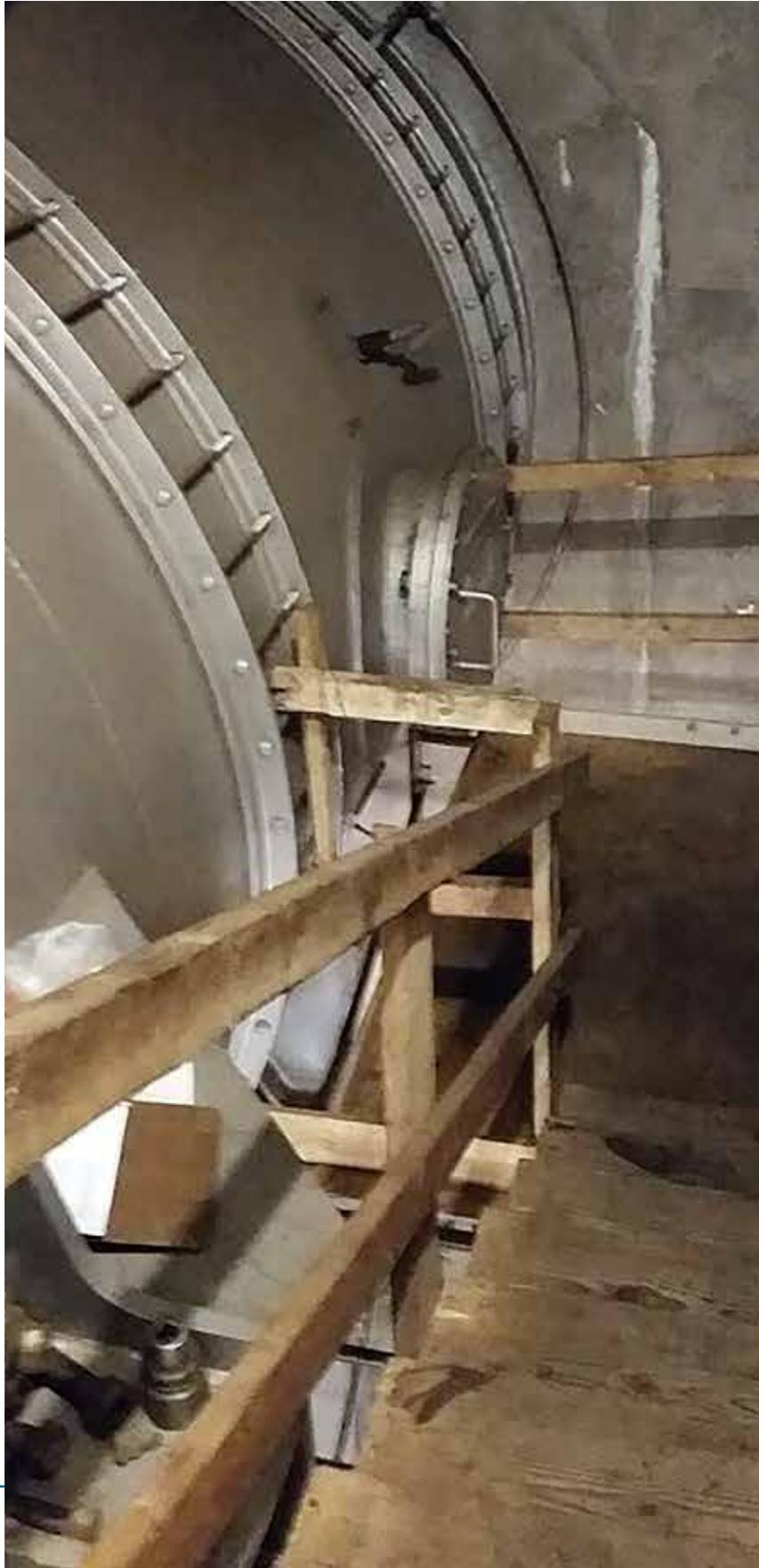
*Photo at right shows an access hole into one of the discharge pipes inside the plant.*
