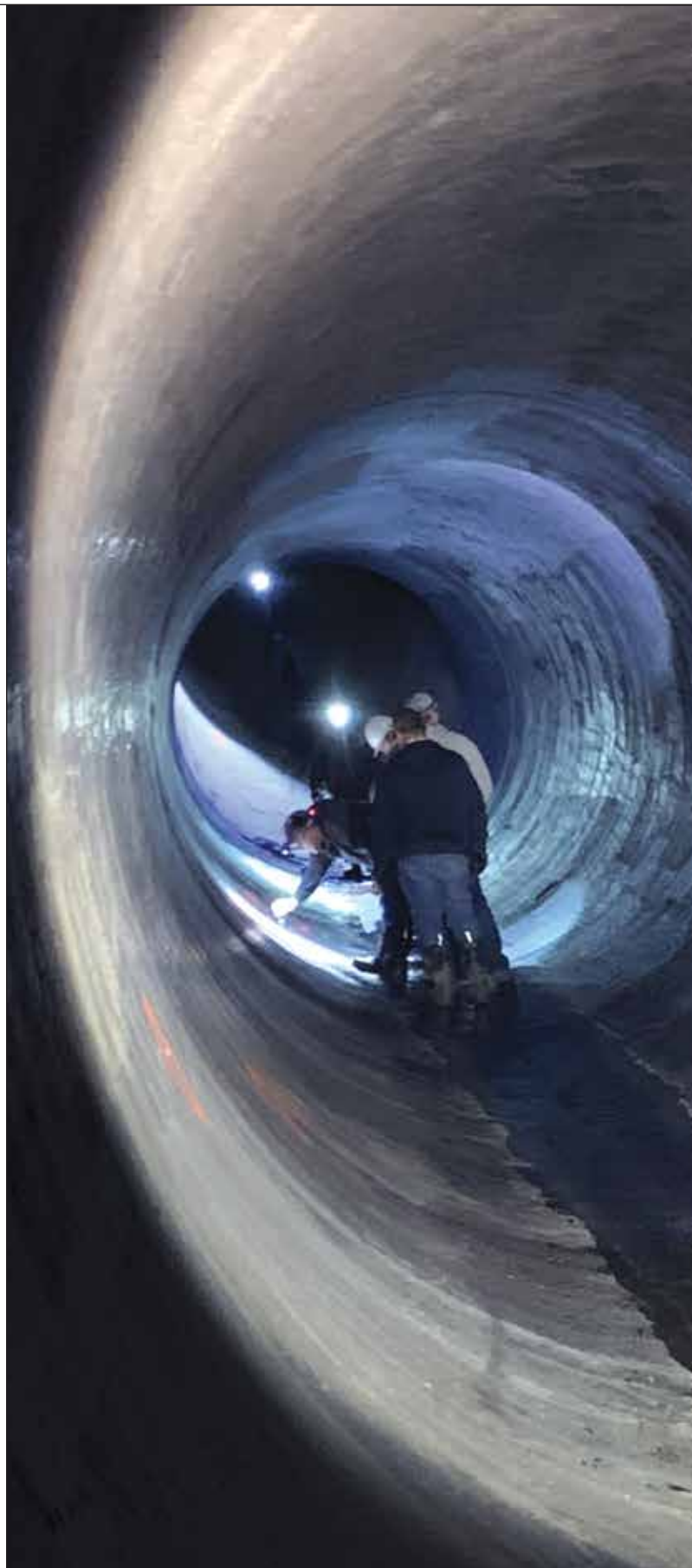
Pre-inspection of tunnel and marking suspect areas.
