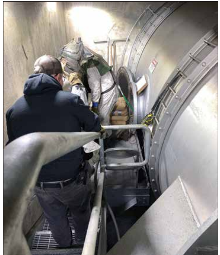
Entering the tunnel via the fourth floor manway.
