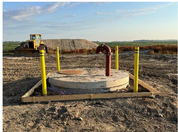
Typical air release manhole
