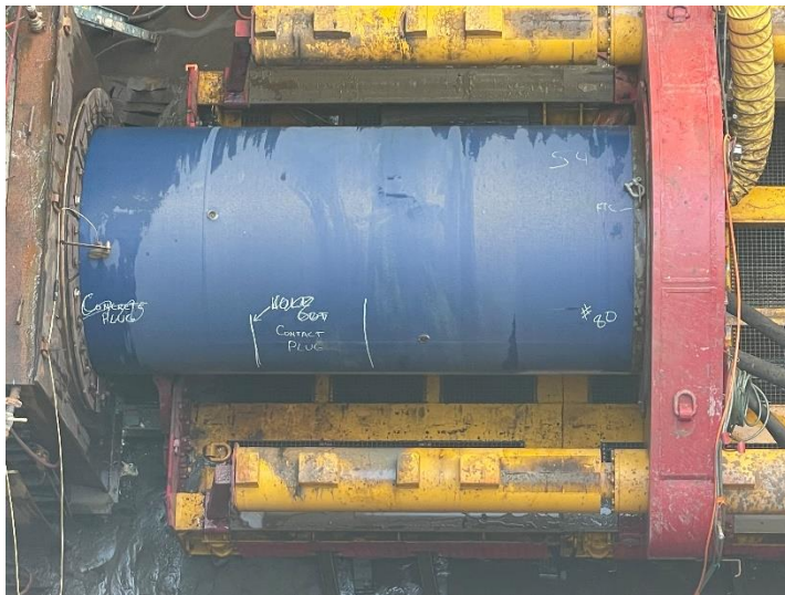
Last pipe being pushed in
