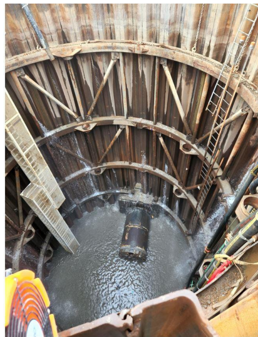
MTBM holing through the coffer dam
