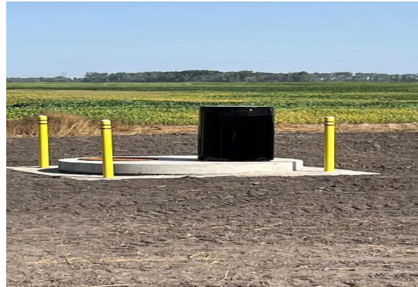
Typical Air Release Manhole
