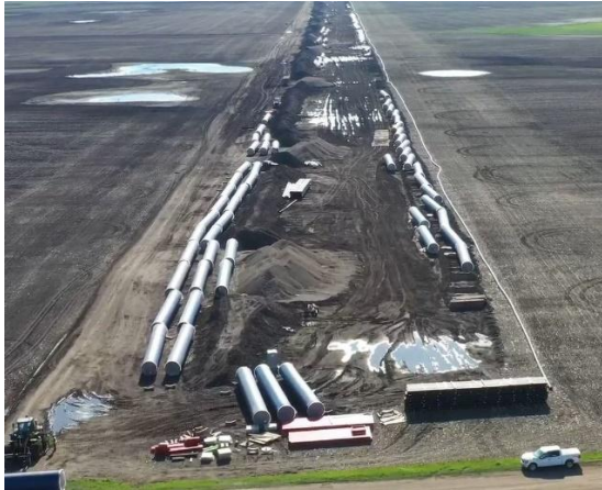
Stored Pipe on Site
