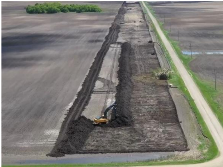
Stripping Topsoil
