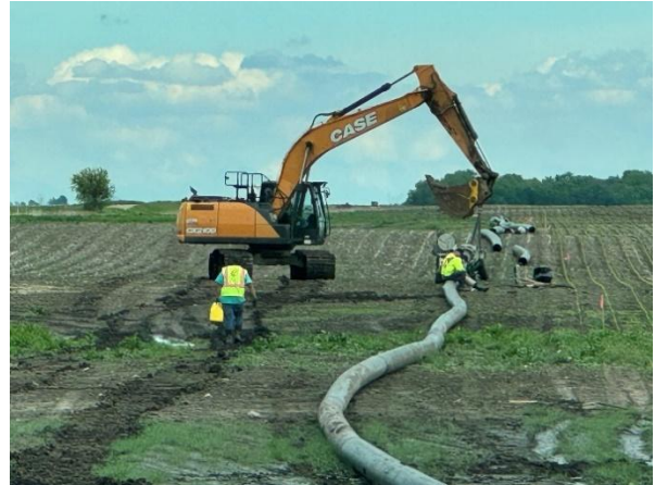
Placing Dewatering Pipe
