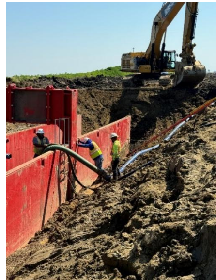
Trench Box w/ Dewatering Pipes
